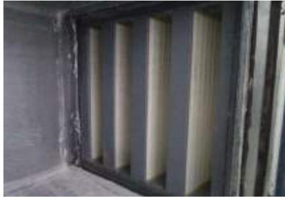
Air filter MVX-E10-03-A-S-D-PG-Y-H23-03 at a differential pressure of about 137 Pa.
